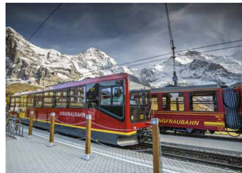
The Jungfrau Railway – the highest in Europe, above; an upgraded gondola, top
